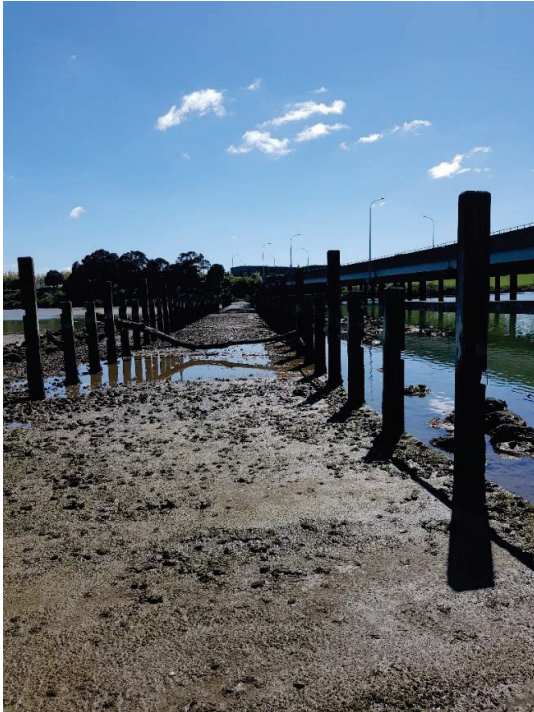
Figure 3: Existing Weir across Ōtara Creek
