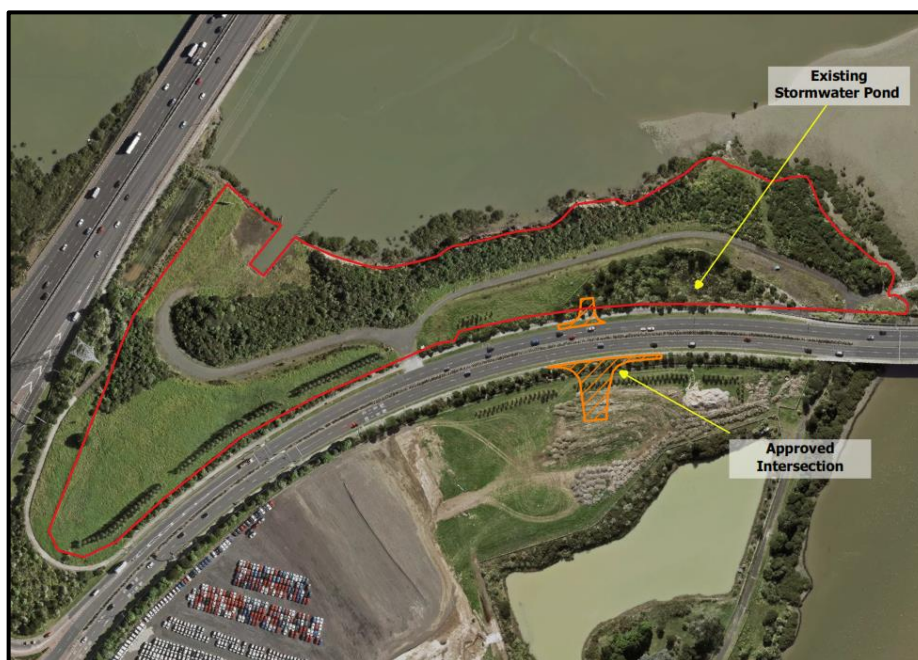
Figure 5-5: Access into the PC area
