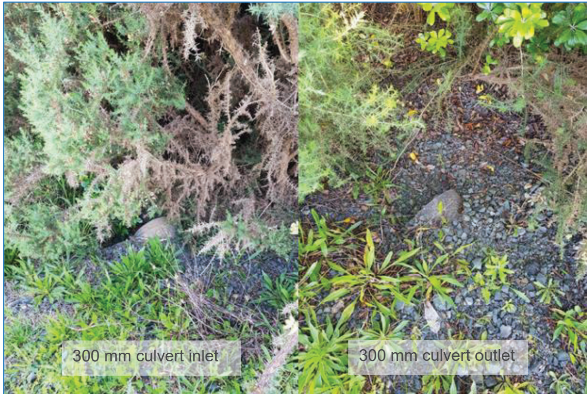
Figure 8: 300mm culvert across the internal gravel road
