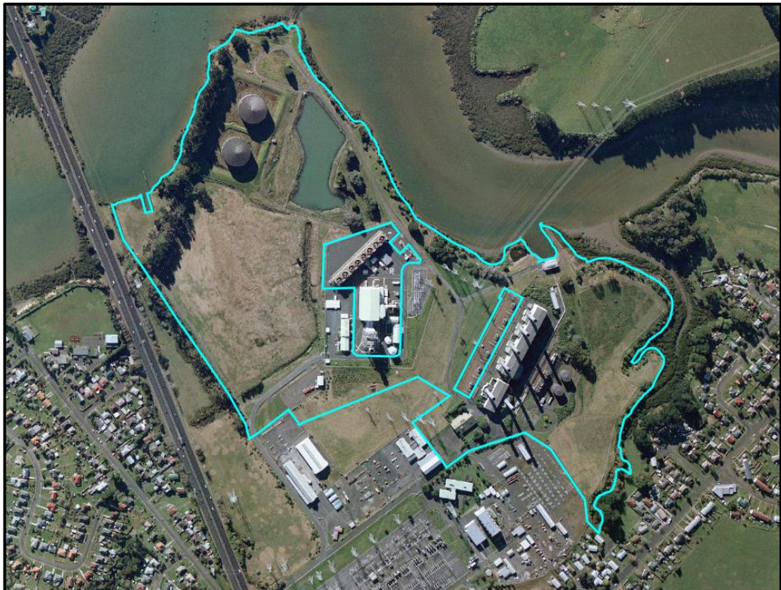
Figure 3-2: Ōtāhuhu Power Station Site in 2001 (Source: Auckland Council Geomaps Aerial Photography 2001)
