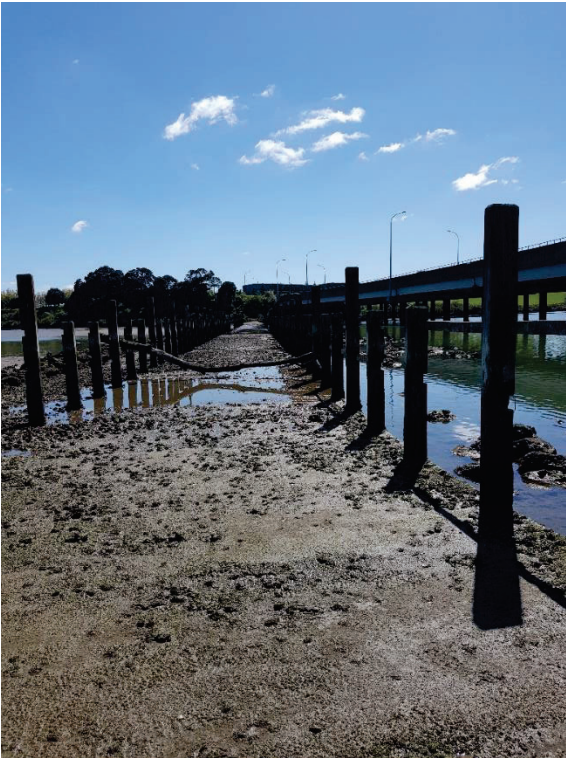
Figure 3: Existing Weir across Ōtara Creek
